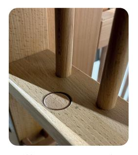
6. Position the wooden plug flush in the opening. Hold it in position if necessary.
