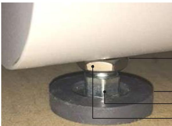
Max. 20 mm between the top of the height adjuster and the round pipe
